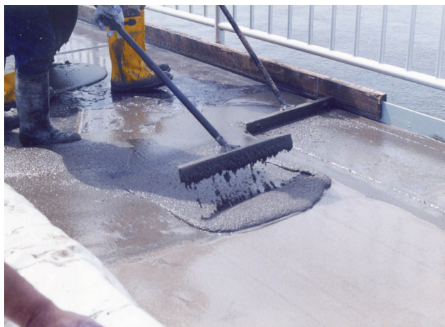
Fig. 6.3.2.1—Application of PC slurry with gauge rakes.
