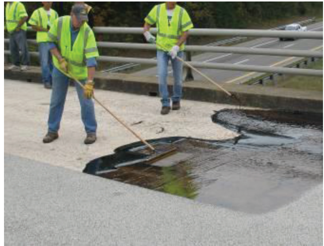
Fig. 6.2.1b—Spreading of mixed epoxy resin with notched squeegees.
