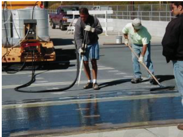
Fig. 6.2.1d—Two-component resin mixed through a static mixing nozzle before application.
