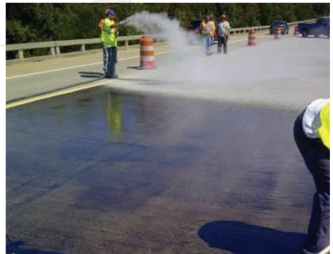
Fig. 6.2.2b—Broadcast aggregate applied with pressurized aggregate tank.
