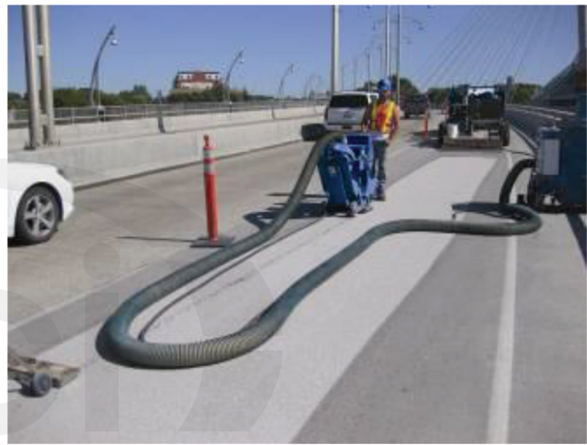
Fig. 5.2.3.1b—Small portable walk-behind shot-blast machine.
