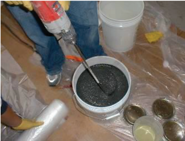
Fig. 6.3.1.1—Mixing of slurry components with drill and jiffy mixer.
