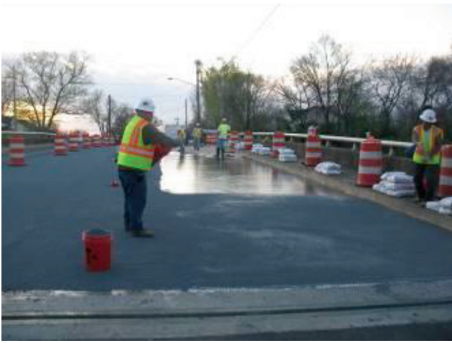
Fig. 6.2.2c—Broadcast aggregate hand applied.
