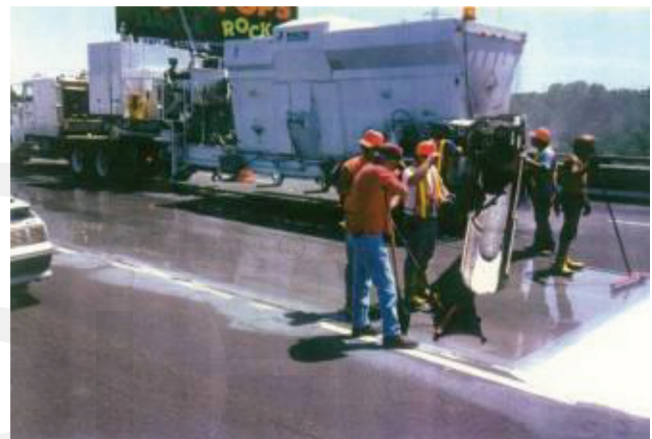
Fig. 6.3.1.3—Mobile continuous mixing truck.
