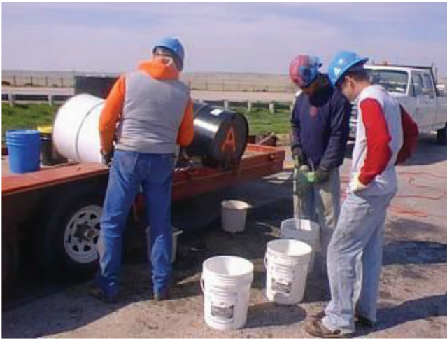
Fig. 6.2.1a—Mixing of two-component epoxy resin with drill and jiffy mixer.
