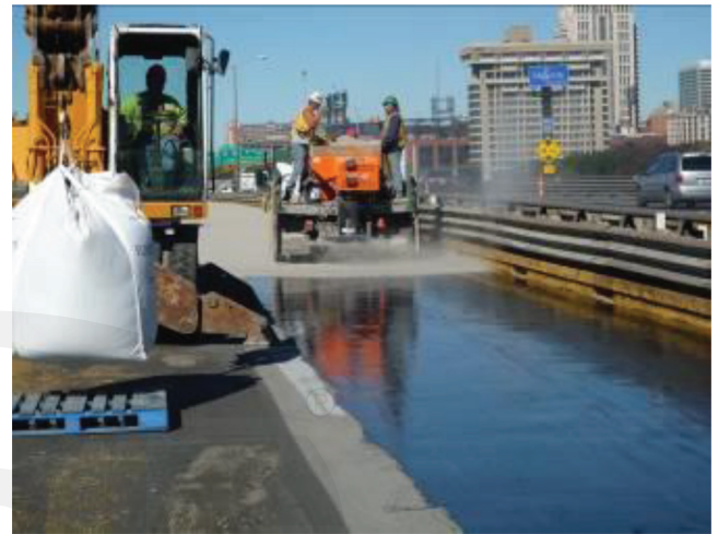
Fig. 6.2.2a—Broadcast aggregate applied with truck-mounted chip spreader.
