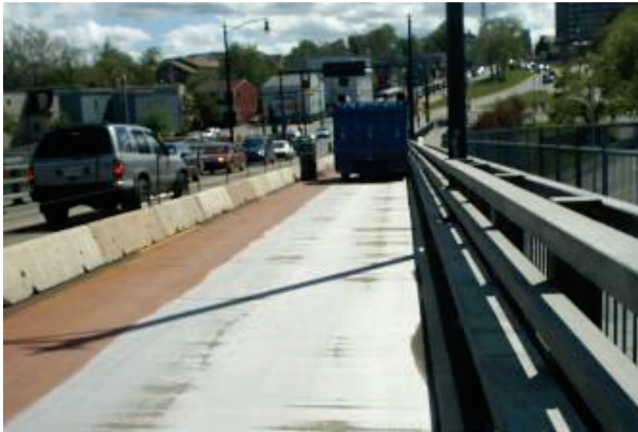
Fig. 5.3—Steel orthotropic bridge deck after shot-blasting.
