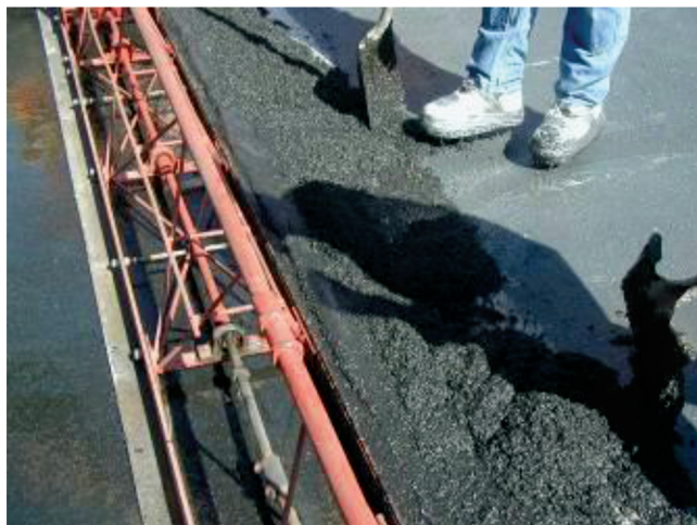
Fig. 6.3.2.2—Application of premix PC overlay with vibratory screed.
