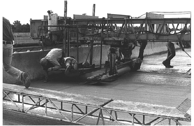
Fig. 4.29—Double roller finisher.
