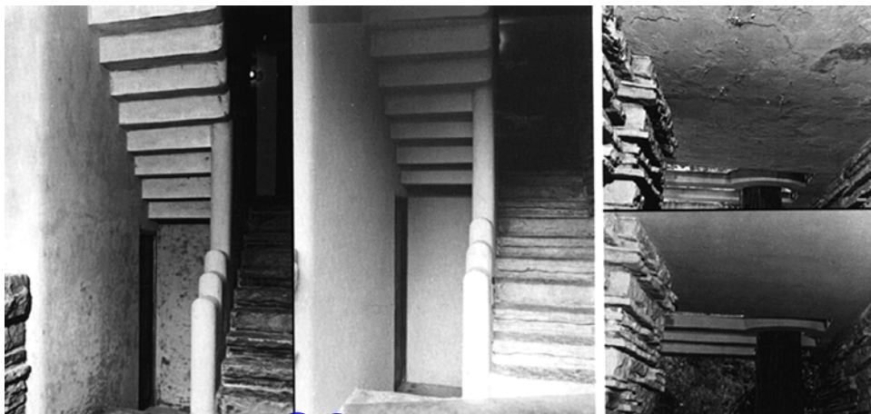
Fig. 4.45—Spalled concrete restored with an acrylic latex-modified patching mortar.
