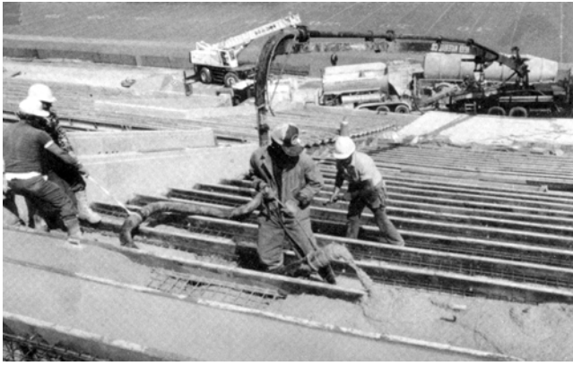
Fig. 4.28—Pumping LMC.
